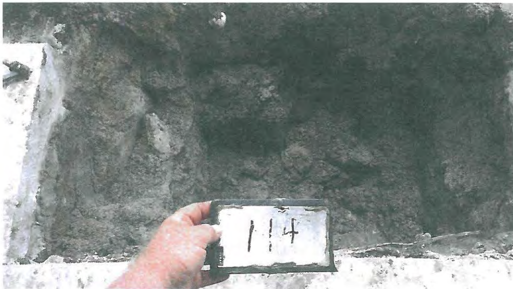
Picture 2: UST 114Banyan excavation.
